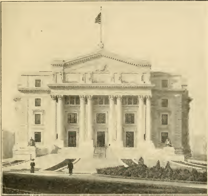
ESSEX COUNTY COURT HOUSE, MARKET, 13th AVENUE AND HIGH STREET COST OF LAND, $126,768.05; BUILDING, $1,821,136.86
